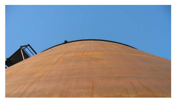
Corrosion can be defined as the deterioration of material by reaction to its environment. Water intrusion is the principal cause of corrosion problems encountered in the field use of equipment. At normal atmospheric temperatures the moisture in the air is enough to start corrosive action. Oxygen is essential for corrosion to occur in water at ambient temperatures. Other factors that affect the tendency of a metal to corrode are:
