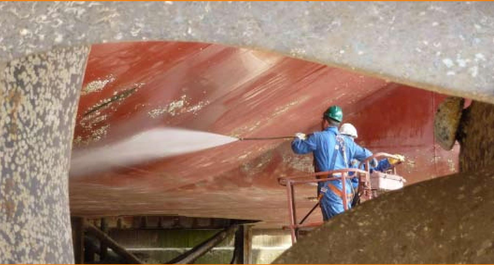
Some applications require cleaning with water, or ultra-high pressure cleaning which can remove loosely adhered rust or previous coatings.
