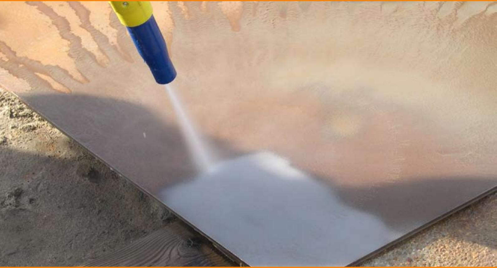
Slurry blasting is a technique for cleaning surfaces with a mixture of fresh water and abrasive where the elimination, or control of abrasive dust is required.
